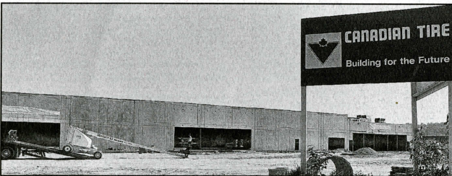
New commercial construction.
